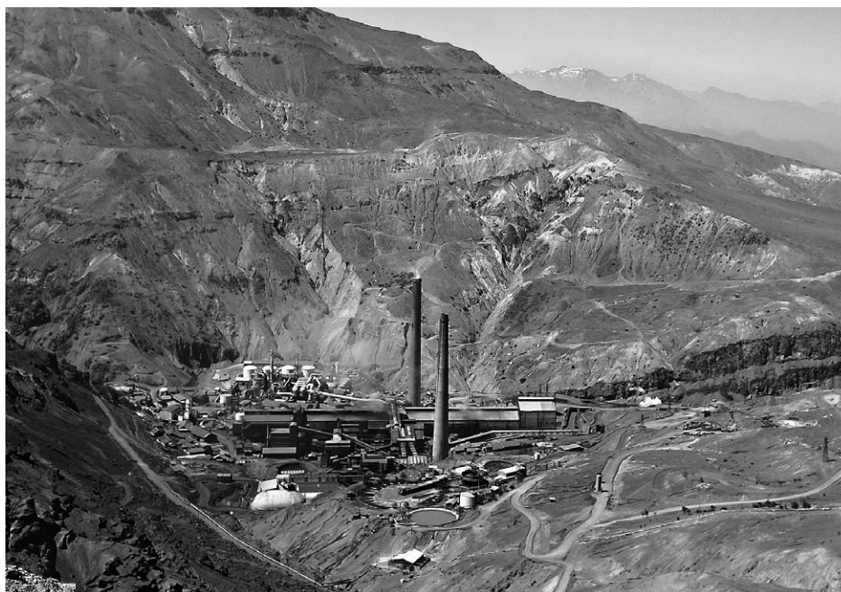
Copper mine in Chile Photo: Frank Jakobi
